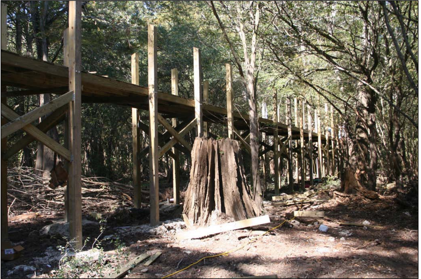
An example of the boardwalk nearing completion at Sky Lake WMA. Note the old cypress stump, probably from when the swamp was originally logged decades ago. This stump is about 6 ft tall, and the boardwalk looks like it will be 8 to 10 ft above the ground along most of its route. Photo by Don C. Bragg.
