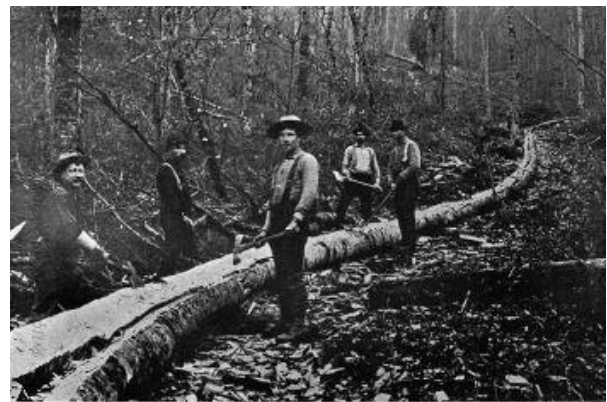
Figure 21: Constructing a log slide near Corbett, Pennsylvania (Shoemaker 1914).
